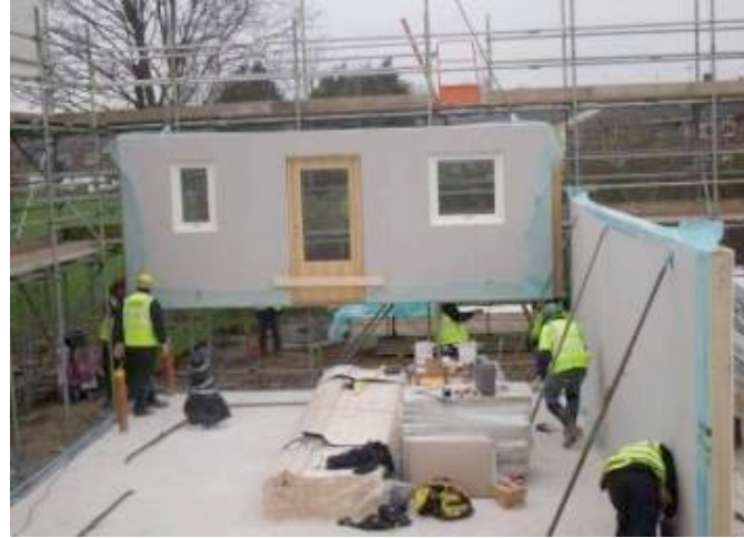
Day 4: Prefabricated panels are lowered into place
