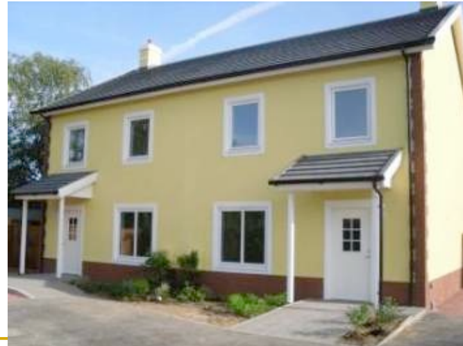
Day 55: Complete; No defects
