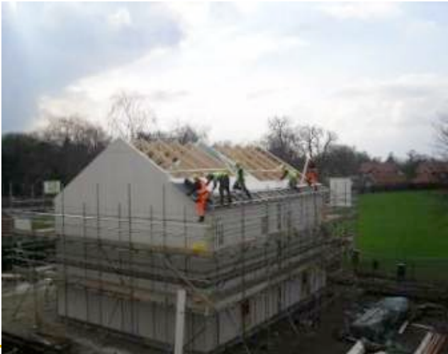
Day 6: Installing roof insulation
