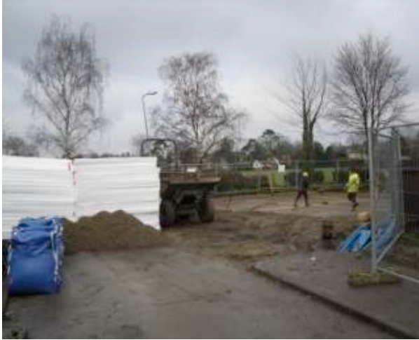
Day 1: Preparing to apply under-floor insulation
