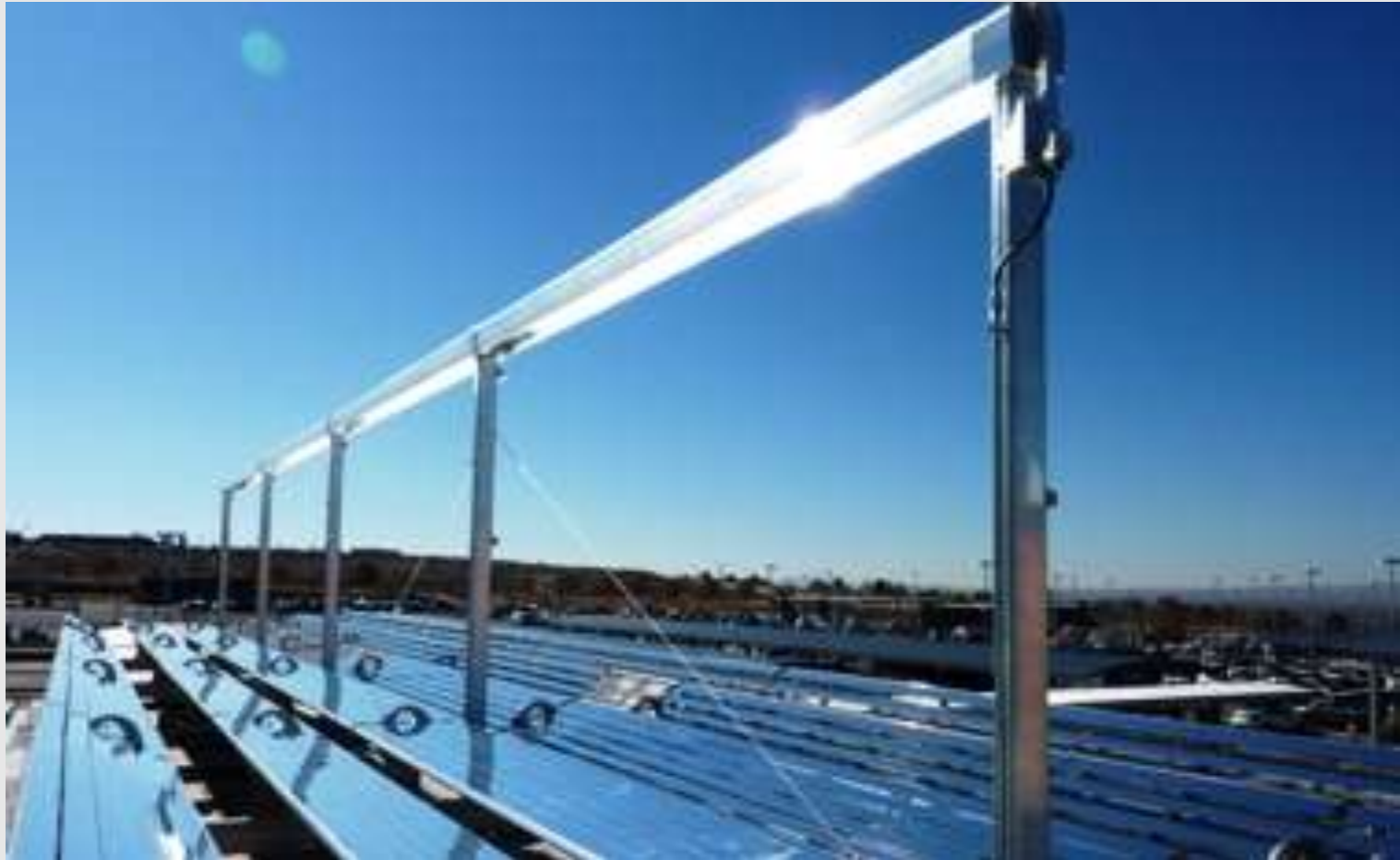
HelioDynamics – Linear Fresnel mirror PV / Thermal hybrid – 10x, 16x.
