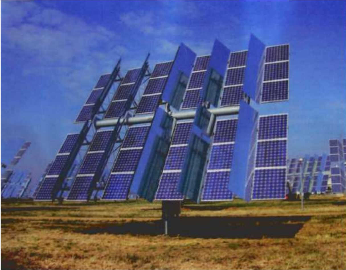
Smoke and mirrors: Solúcar Energía completed this 1.2 MW 2.2x system near Seville in 2006. It is the largest low-concentration PV plant built since Arco Solar's 6 MW 2x plant in California in the 1980s, which was later dismantled.
