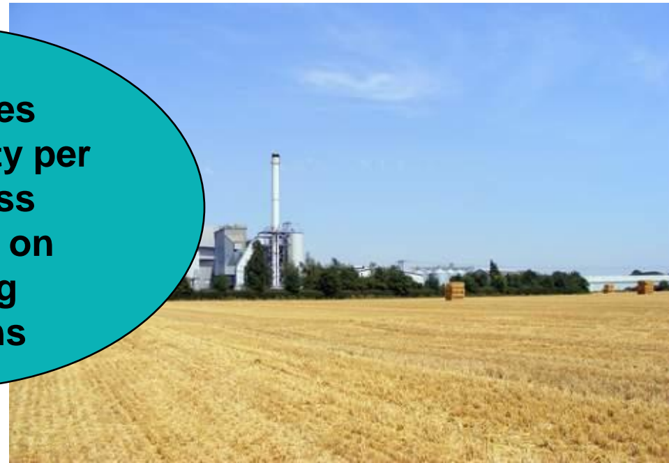
Eye Power Station
