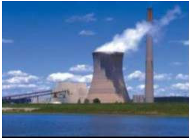
Mountaineer Power Plant
