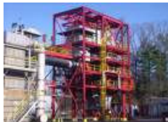
Alstom BSF Windsor US - 15 MWth Oxy - Coals
