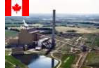
Transalta Canada - >200 MWe Chilled Ammonia - Coal
