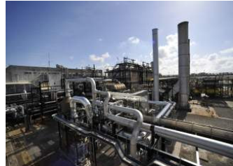
Total Lacq France - 30 MWth Oxy - Gas
