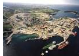
Statoil Mongstad Norway - 40 MWth Chilled Ammonia - Gas
