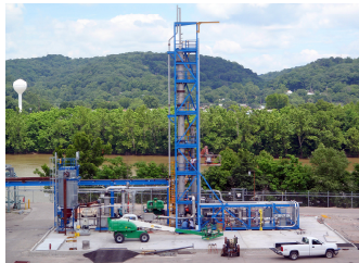
Dow Chemical Co. USA, West Virginia Advanced Amines - Coal
