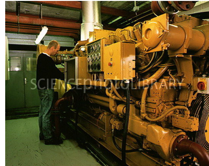
Landfill gas engine and generator at Endersby, Leics. Credit: Martin Bond/Science Photo Library
