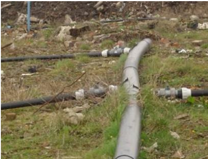
Landfill gas collection pipeline at Summerston Credit: ESRU Strathclyde University
