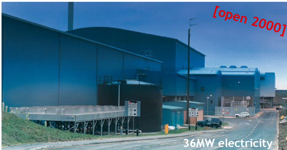
EPR Ely Ltd 36MWe straw fired power station Credit: Fichtner
