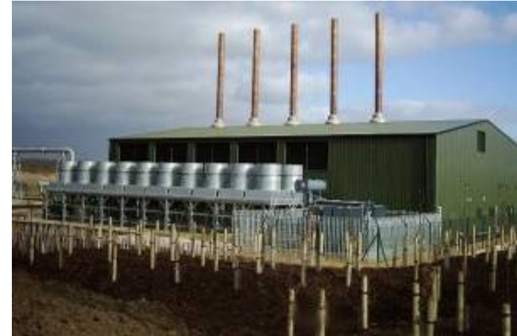
12MW generator plant at Shanks' Calvert Landfill Site near Milton Keynes Credit: Clarke Energy
