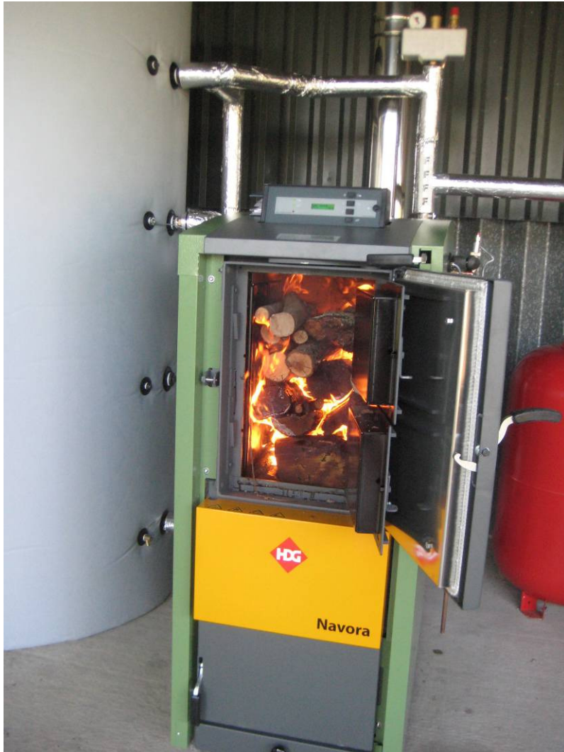
HDG Navora 25kW log boiler installed near Cambridge Credit: Futureneering
