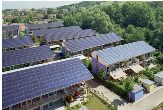
Solarsiedlung (Solar settlement), Freiburg, Germany
